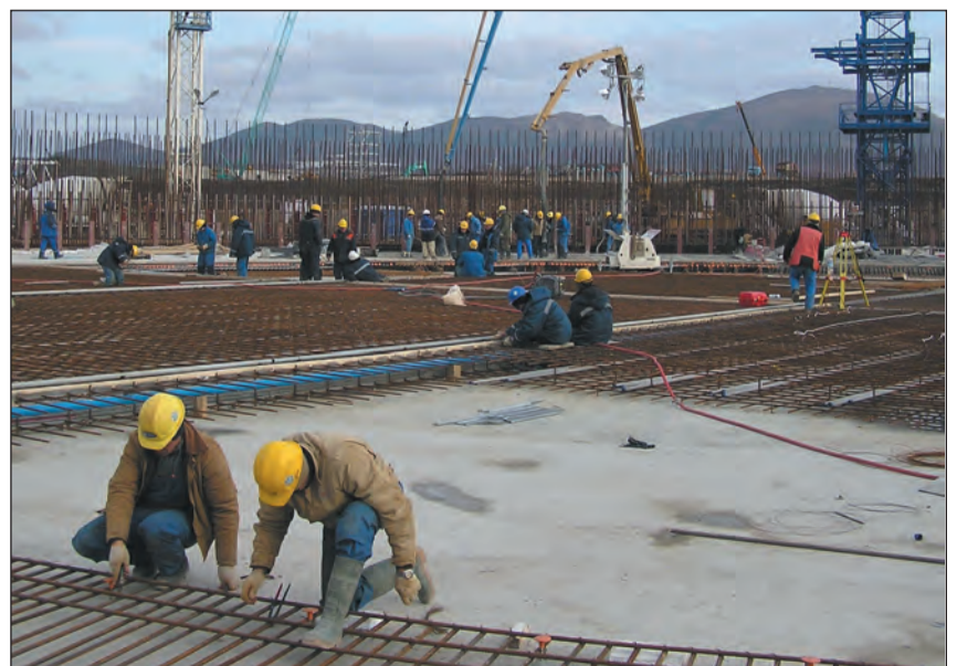
Figure 4: Pouring the slab for an LNG tank on Sakhalin
