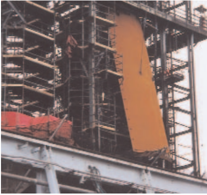
Fig. 5 — Replacement of a vertical section of a coke drum.
