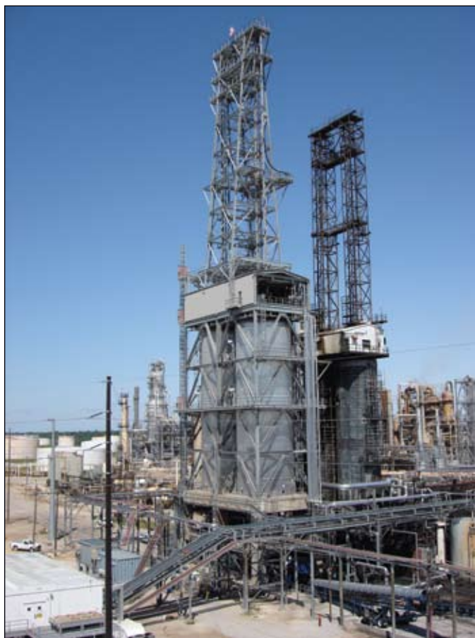
This view shows the completed Frontier El Dorado coker alongside an existing coking structure (Fig. 1).
