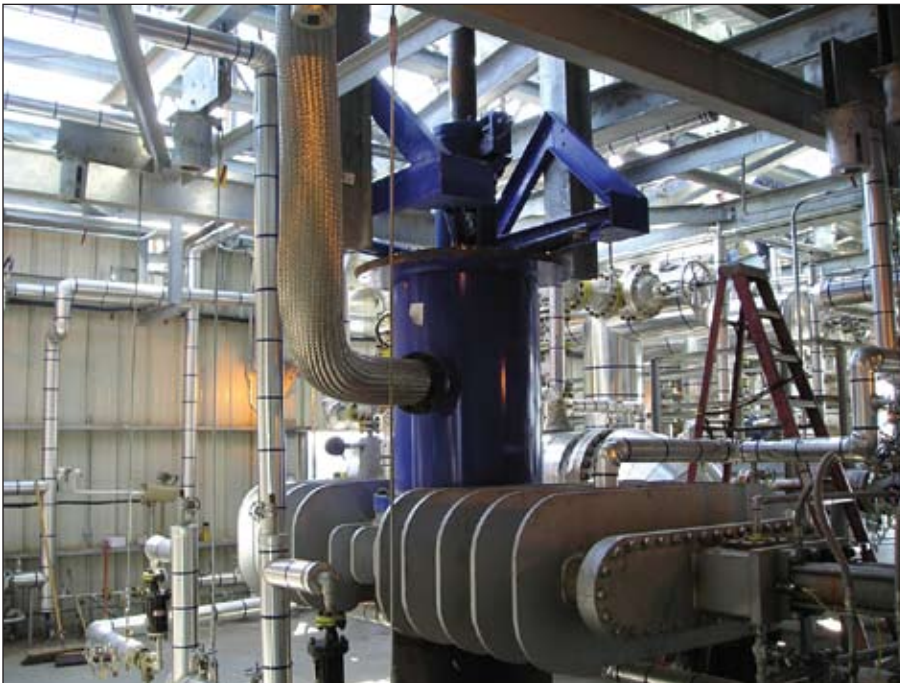
Fig. 6 shows the containment dome with the drillstem parked.
