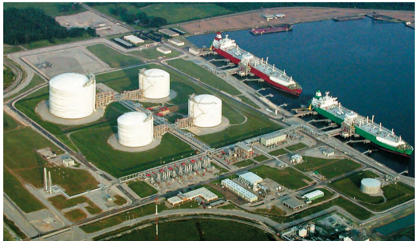
The Trunkline LNG terminal, which was built in 1981, is located southwest of Lake Charles, Louisiana, about 40km (25 miles) from the Gulf of Mexico and accessible to carriers via the ship channel
