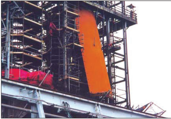
Figure 6 Plate-by-plate replacement method in progress
