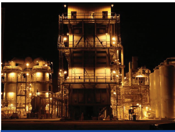
Figure 4. Navajo Refining's cylindrical unit (left) utilised secondary feeds to the PSA. Excess offgas was exported and utilised as fuel for the box reformer (centre).
