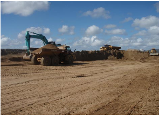
Figure 2. Completion of bulk earthworks for LNG tank at Fisherman's Landing.
